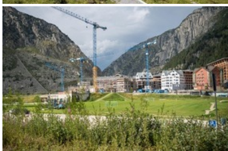
Baustelle Apartmenthaus Frame in Andermatt Reuss © Valentin Luthiger
